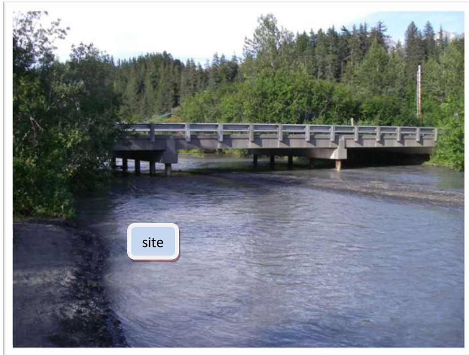
Figure 6.) Salmon Creek at Nash Road looking upstream to in an approximate northeast direction.
